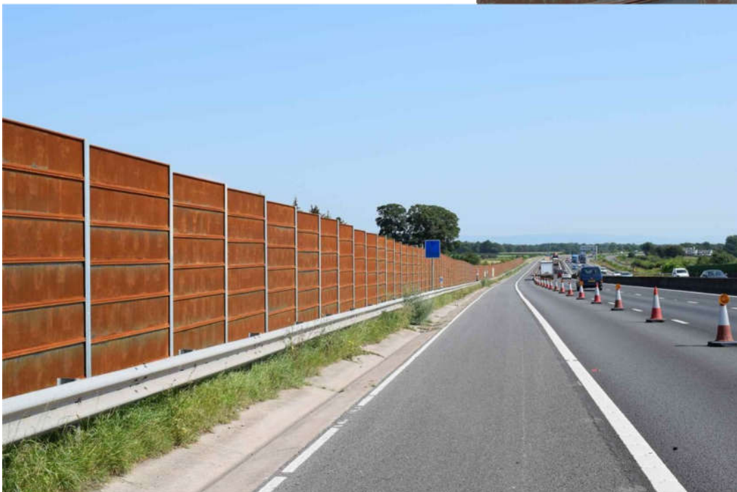
2 Months after installation
